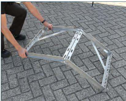
Take out the stainless steel frame, unfold it and put it on the flat surface. Make sure the driving direction is correct.
